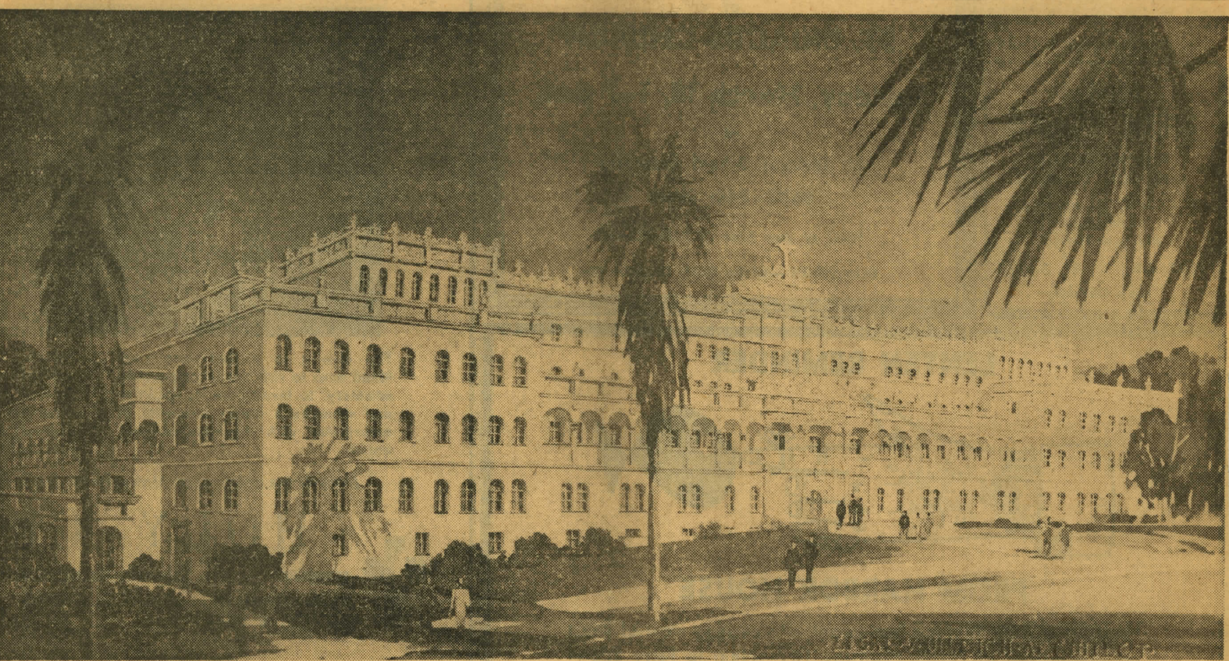
BEAUTIFUL NEW SEMINARY BUILDING—Rapidly rising to its impressive height on the Alcala Park campus is the beautiful Immaculate Heart Seminary Building. The framework is nearing completion on the top floors, and work-
