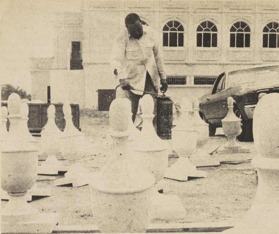
ARMY OF 'PAWNS' —A workman outside the new nursing school building nearing completion on the campus of the University of San Diego sprays a bonding agent onto plaster urns resembling giant chess pieces. The urns will eventually adorn the roof of the building.—SC photo
