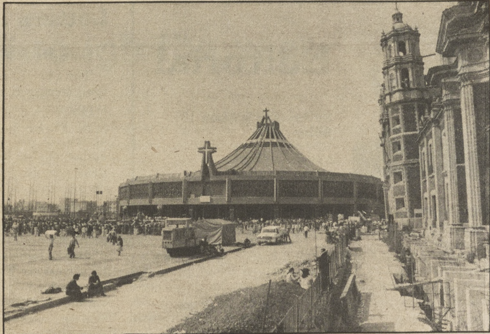
NEW AND OLD — The modern Basilica of Our Lady of Guadalupe is a sharp contrast to the early 18th-century basilica on the right, which is now empty as it cracks and sinks into the dry lake bed which underlies Mexico City. Extensive work is going on to save the structure.
