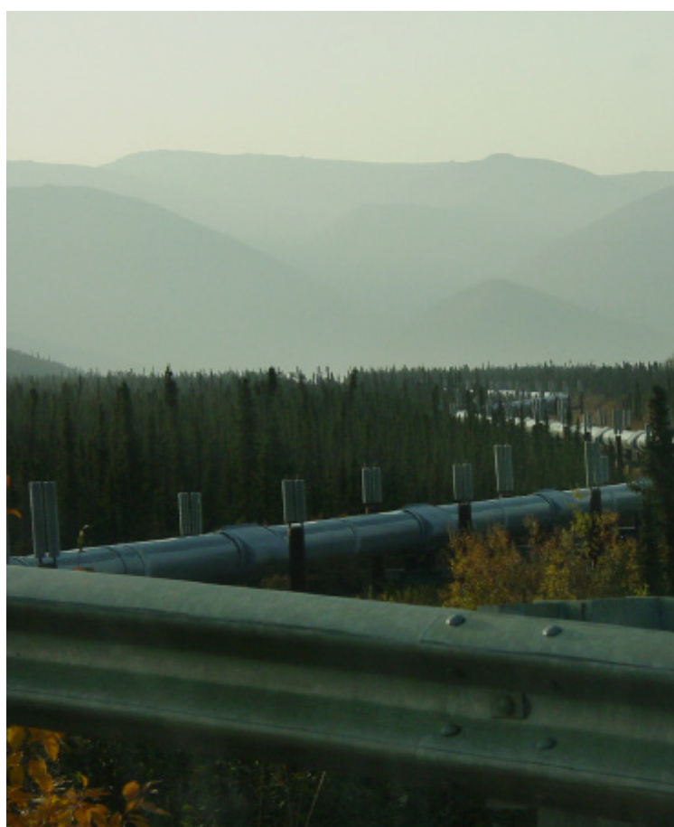
The Alaskan Pipeline outside of Fairbanks, Alaska.
